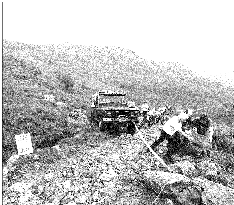
Winch power helps man power – volunteers rebuild Garburn Road
