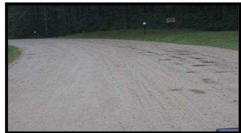
**Example of proper crown slope at left only and flat at right, with potholes; same road, different slope on each side**
