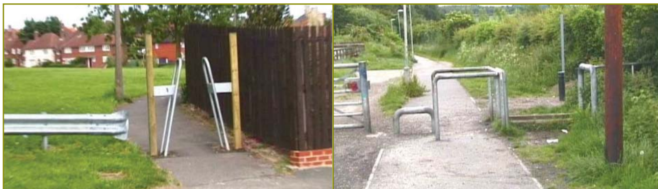
Examples of how to discourage illegal activity from accessing specific rights of way
