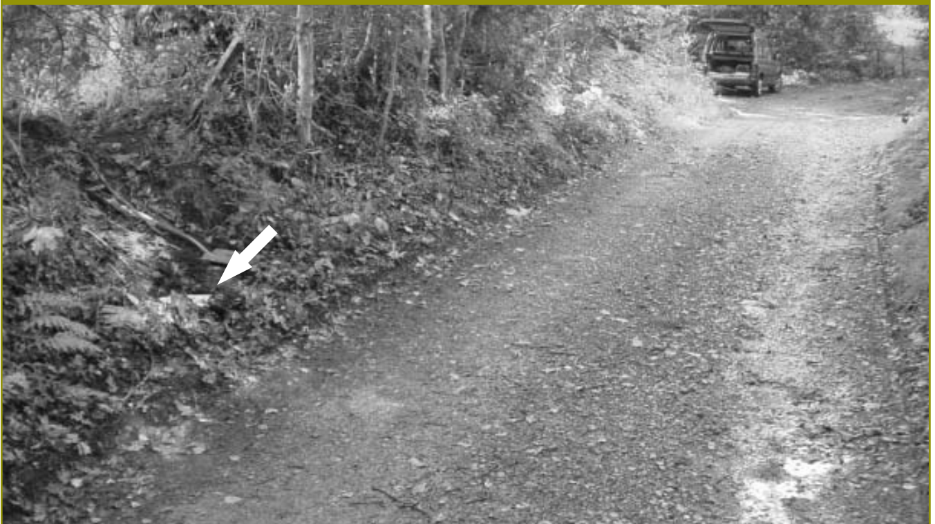
Figure 2.1b: Duddon Electronics vehicle logger installed but not covered with soil
